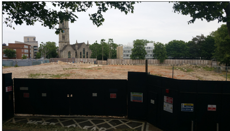
Figure 8: The demolished Bacton low-rise estate standing empty for nearly a decade
